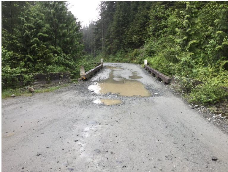
Approach from Left Bank when facing downstream
