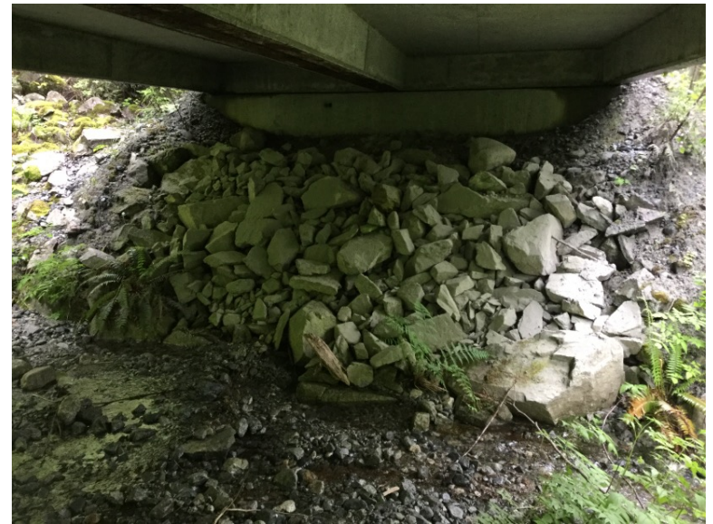
Left Bank Abutment when facing downstream
