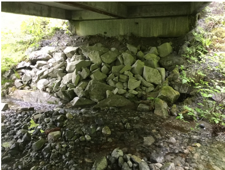
Right Bank Abutment when facing downstream
